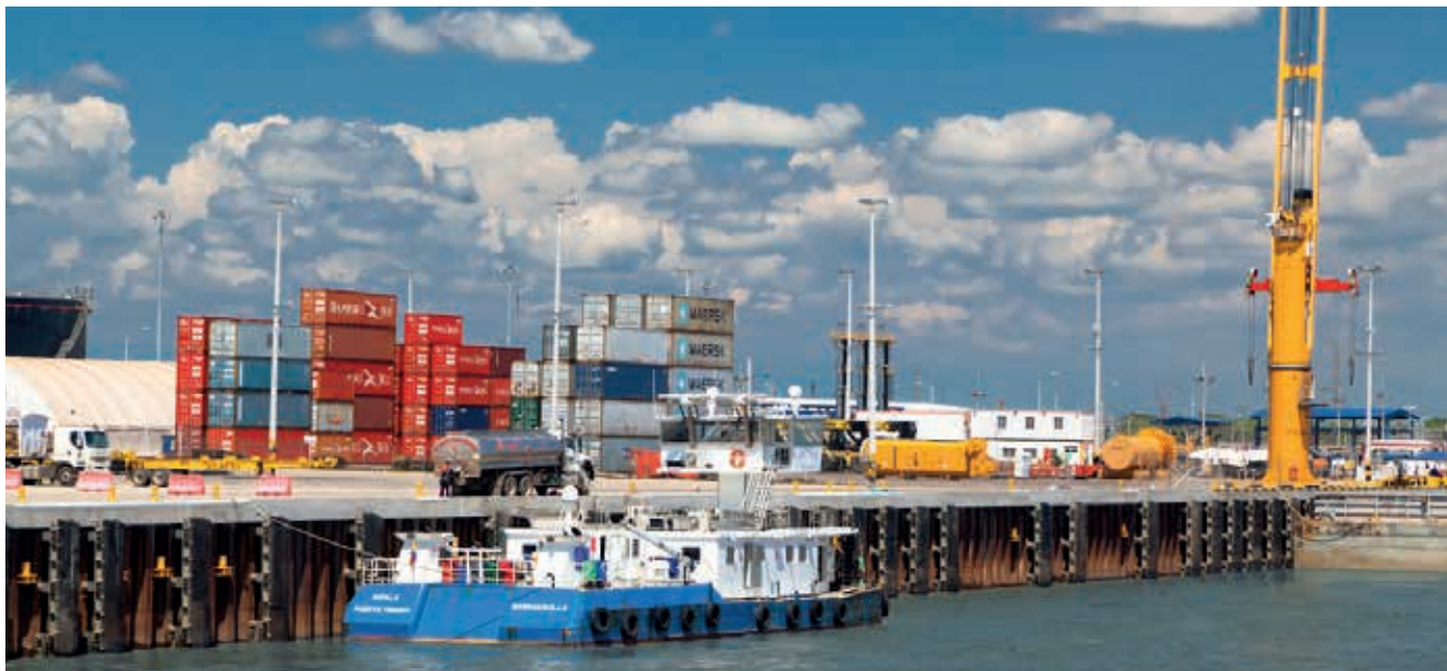
Impala Terminal's inland riverside port on the Magdalena River at Barrancabermeja, Colombia.
