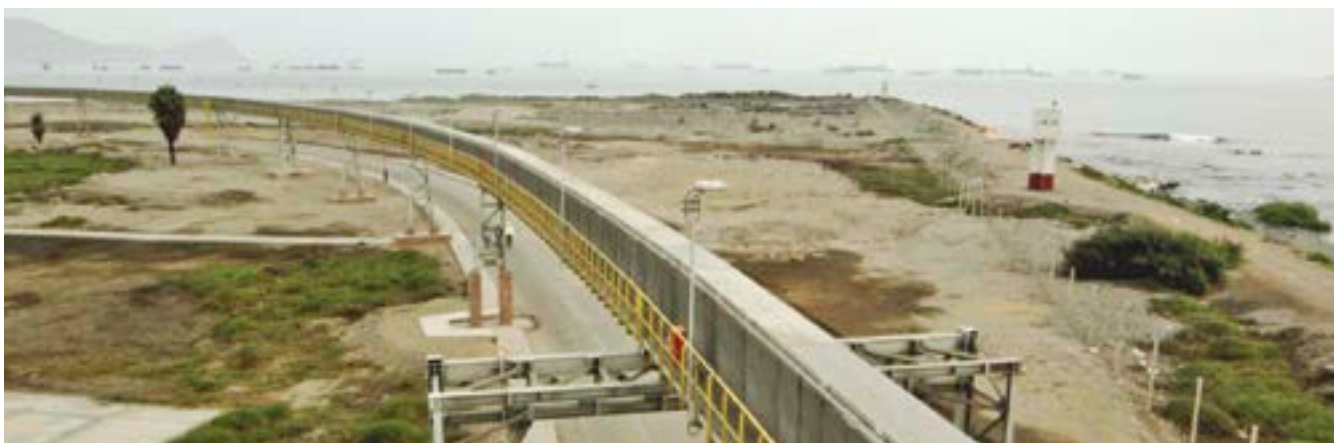
Impala Terminals' jointly owned covered conveyor belt expansion at the Port of Callao, Peru.
